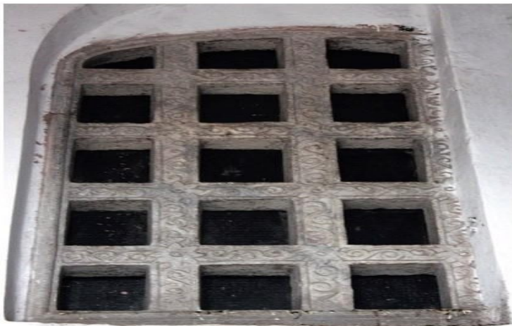
Fig.4 Window transenna in the passage to the Baptistery (photo R. Flaminio)
